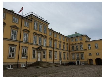
Facader mod gårdrummet.
